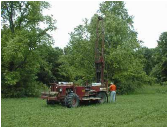
Figure 1. Off-road drill rig.
