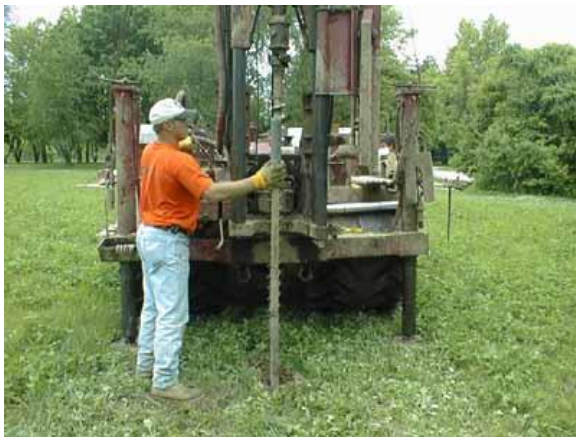
Figure 3. The operators uses the auger to drill down to the first sampling depth. Soil pulled out of the hole is noted so that the driller can approximate the depth for each change of soil type.
